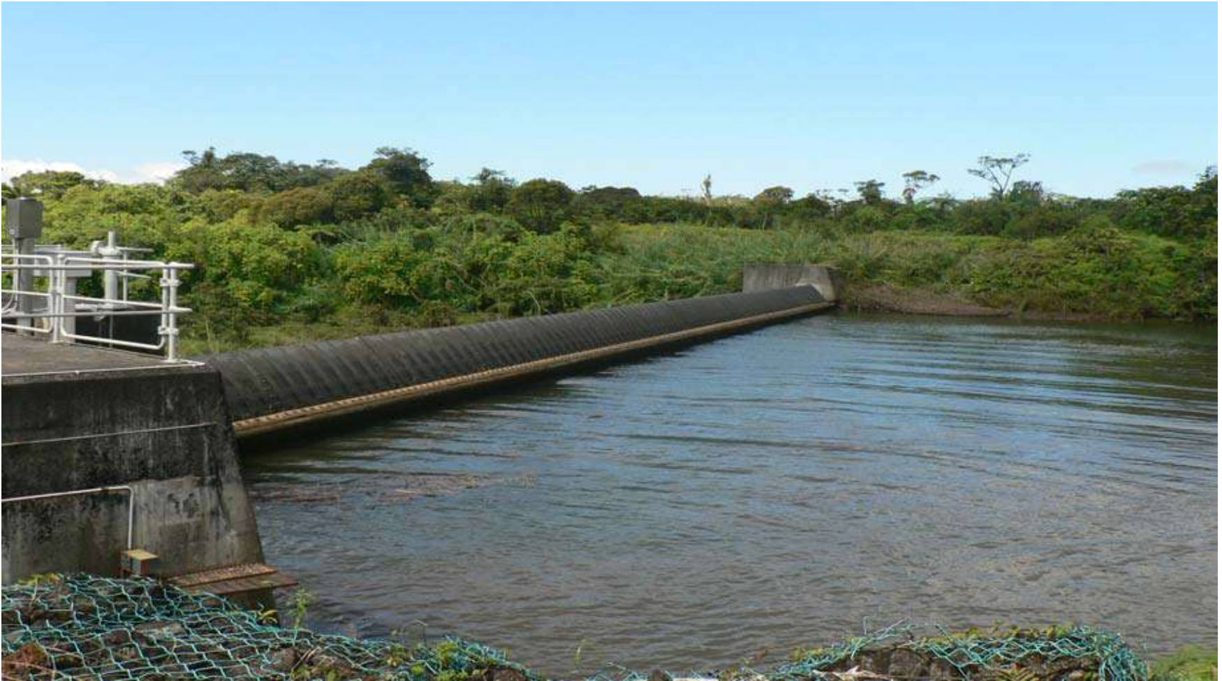
Pictures of Existing Wainisavulevu Weir
