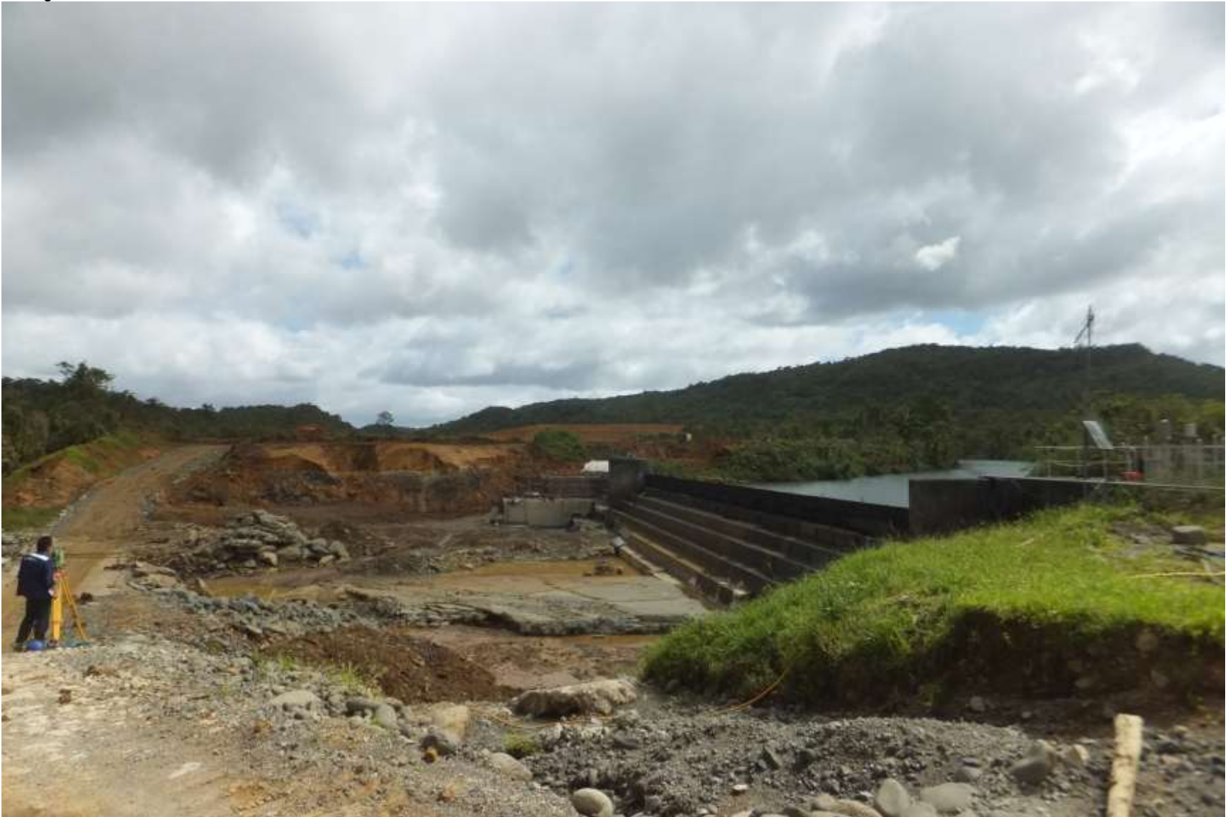
During Construction Pictures:
