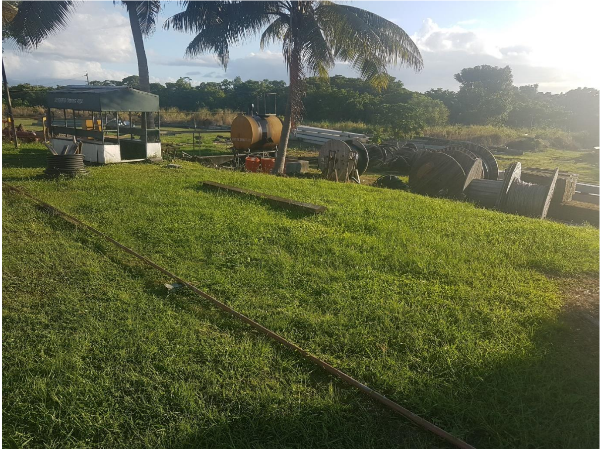
Figure 1 Site for new Lube containment bund
