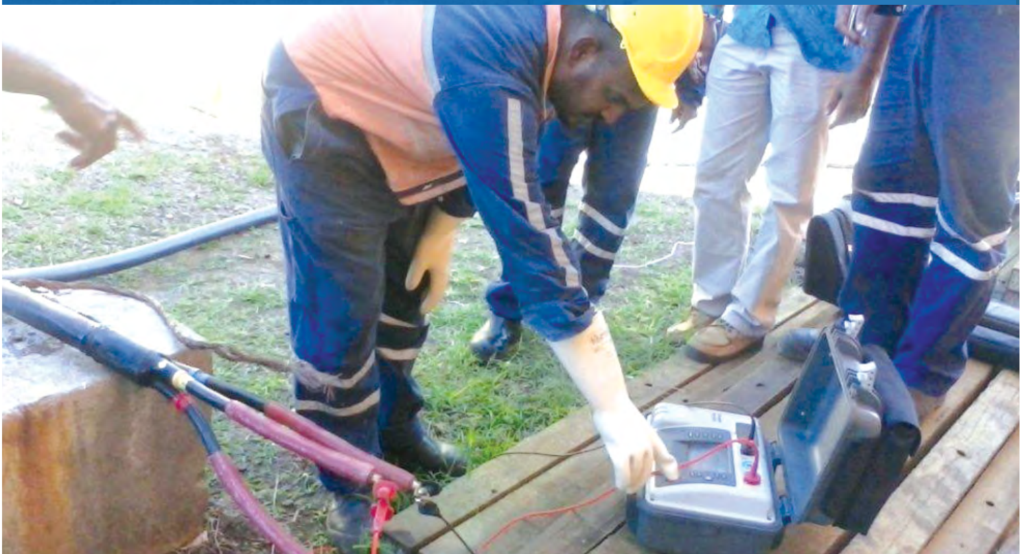
FEA employee carrying out the testing of new cables before being commissioned by the FEA technicians.
