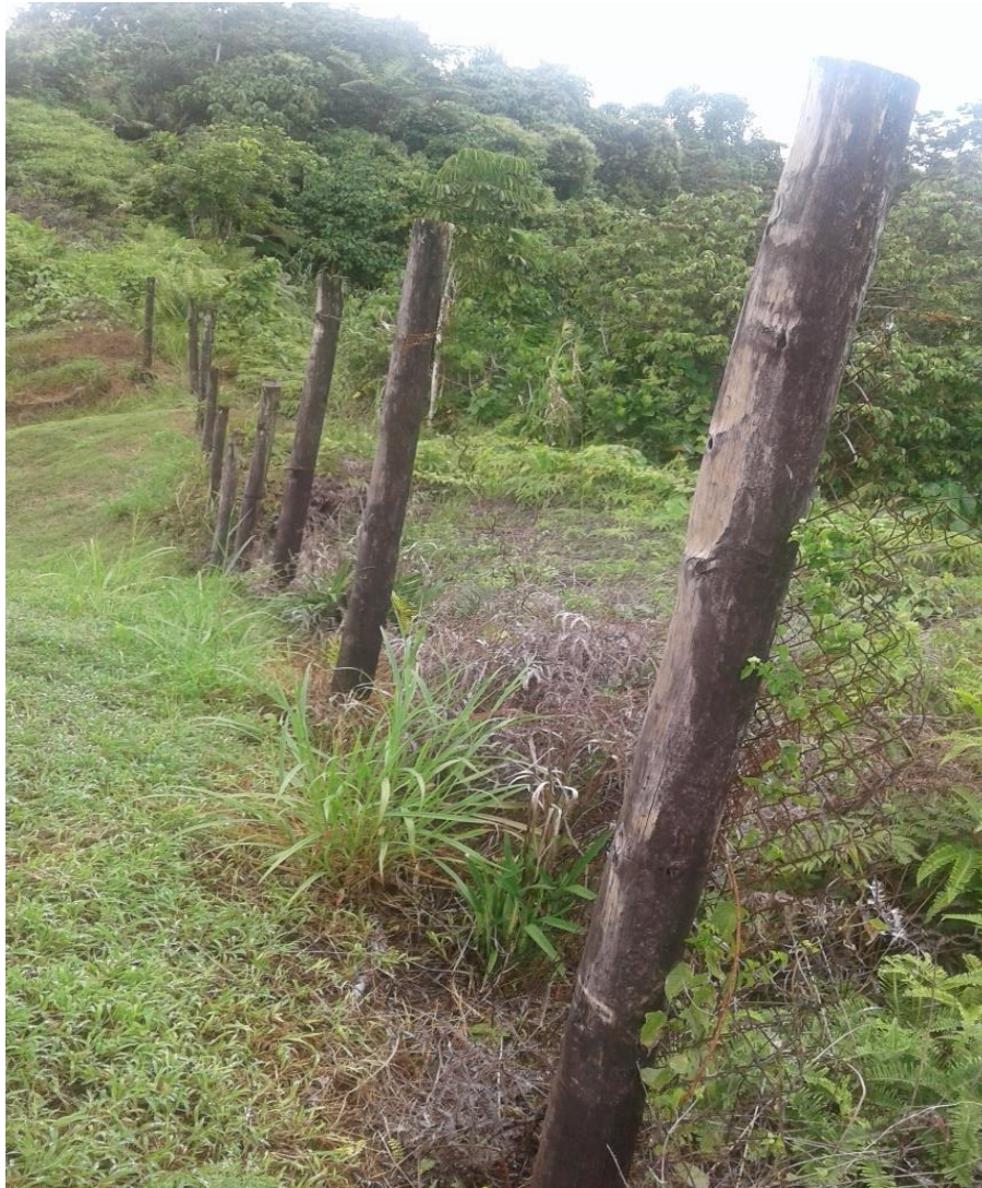
Fig 3. Section of fence where chain link is missing
