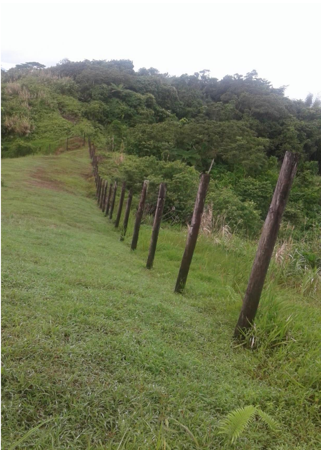
Fig1. Section of fence where chain link is missing
