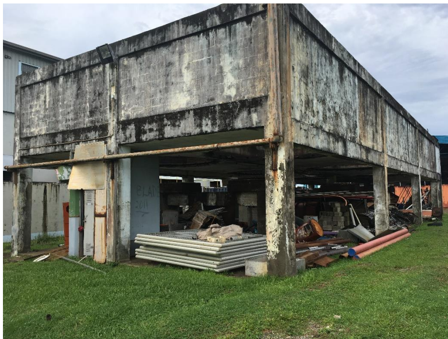
Figure 1 Site Photo of the Building
