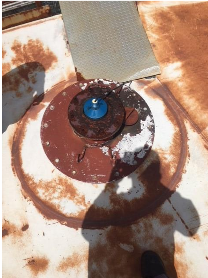
Figure 5 shows the Sensor housing which is located at the top of the Fuel Tank.
