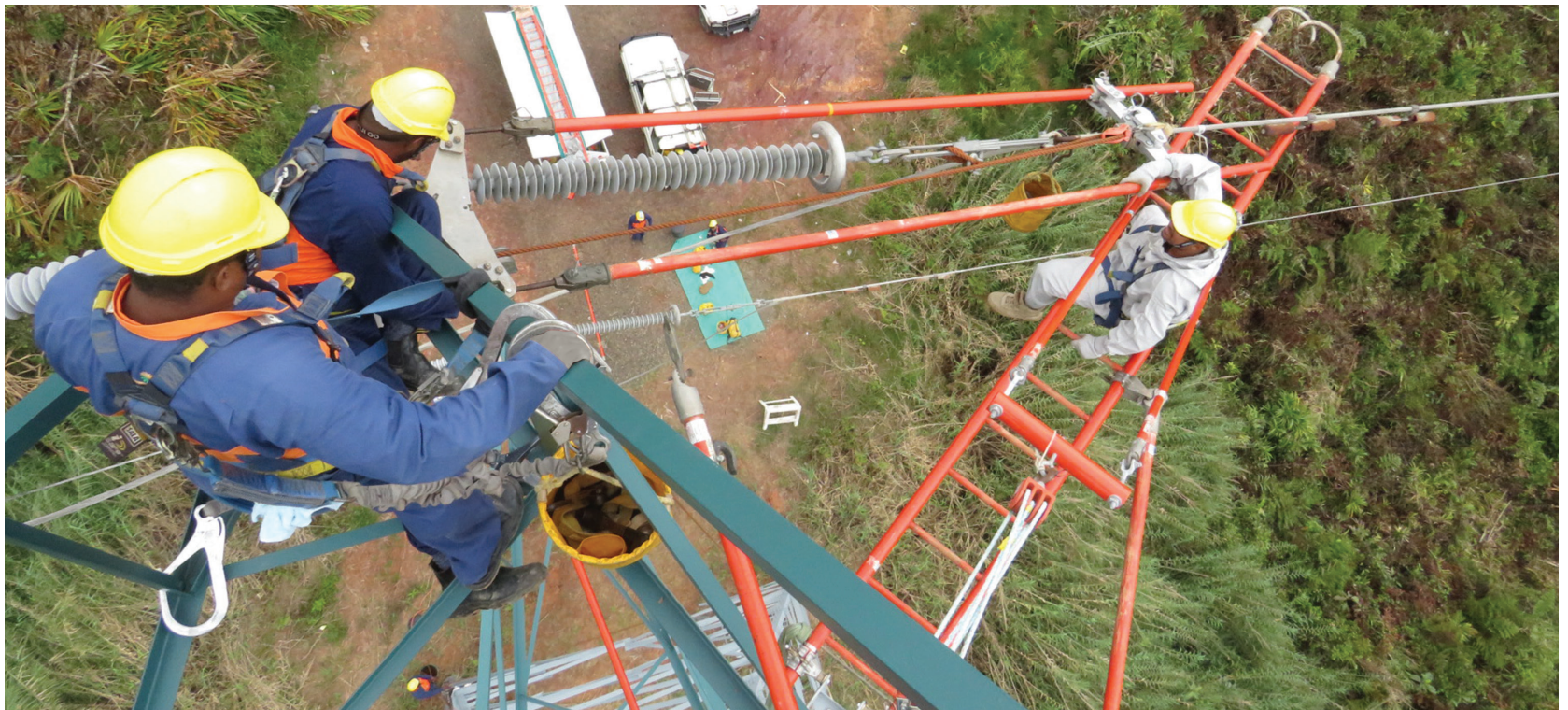
EFL network line mechanics carrying out live-line maintenance on the 132,000 volts transmission line without putting off the power supply to our valued customers.
