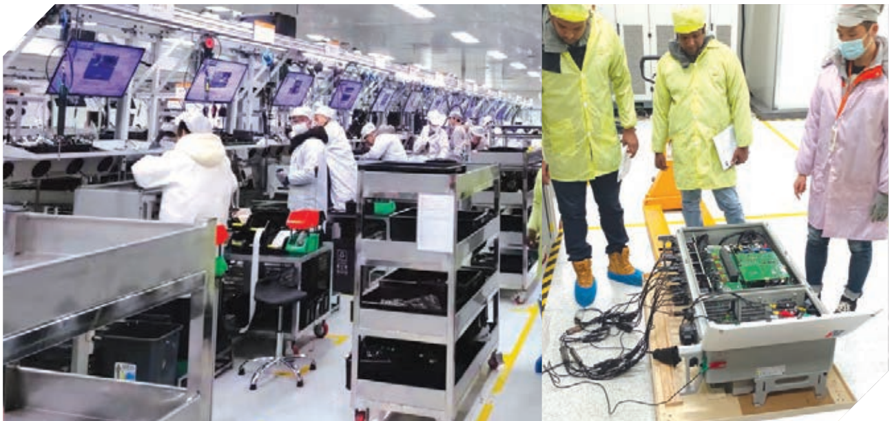
The EFL Project Electrical Engineer and Acting Manager Civil attend the factory acceptance test for SMA string inverters at China for 1MW Taveuni Solar Farm.
