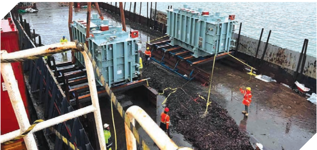
EFL imported new power transformers to replace existing aged power transformers to increase the reliability and security of power supply to its customers.
