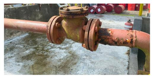
Figure 2: 3" fill line and non-return valve
