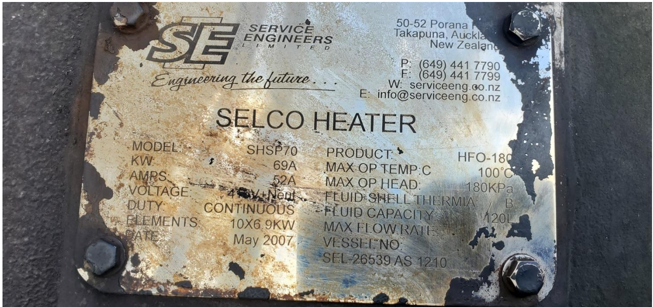
Figure 2: Existing Heater Name plate
