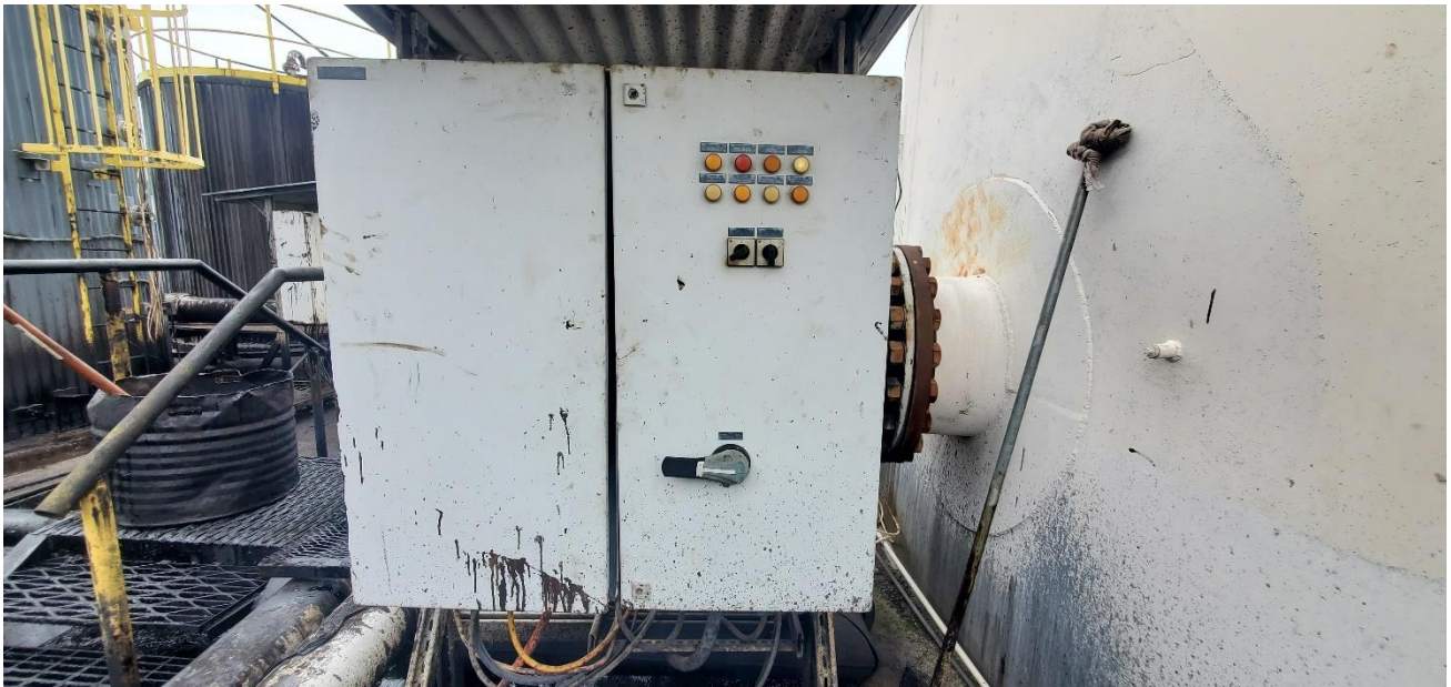
Figure 3: Existing Heater Control Panel
