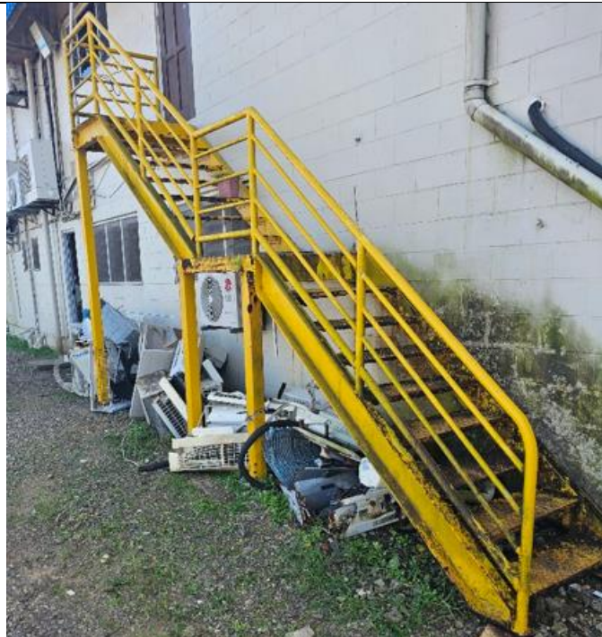
Pic of existing stairway - for illustration purpose only
